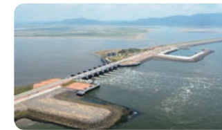
Garyeok drainage floodgate and tourism zone, Saemangeum-Gunsan
