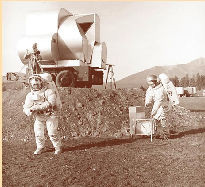
Field testing at Cinder Lake Crater. Flagstaff USGS geologists, acting as astronauts, tested the simulated Lunar Module for future training exercises.
