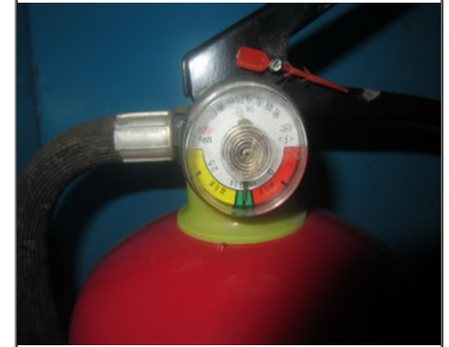
Photo of the inside of the main production hall Fire Extinguisher pressure.JPG
