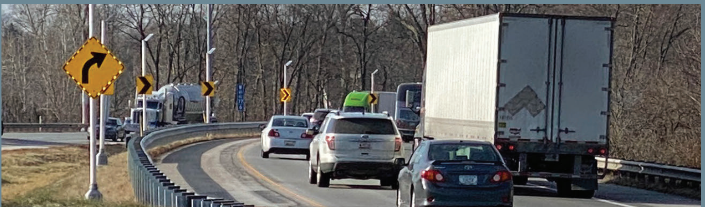
New curvature signage installation at South Bend.
