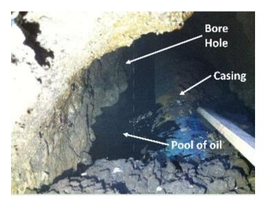
Figure 23: View at the borehole entrance accompanied by audible fluid sounds emanating from the opening
