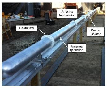
Figure 9: Installation of the dipole antenna
